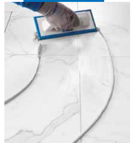
Spreading Ultracolor Plus on marble-effect porcelain floor tiles with a rubber float
