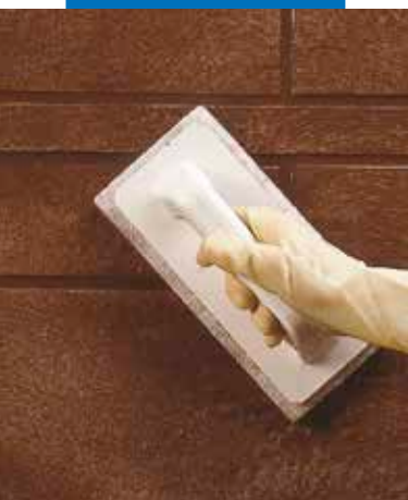
Cleaning the joints with Scotch-Brite® (when the product is partially set)
